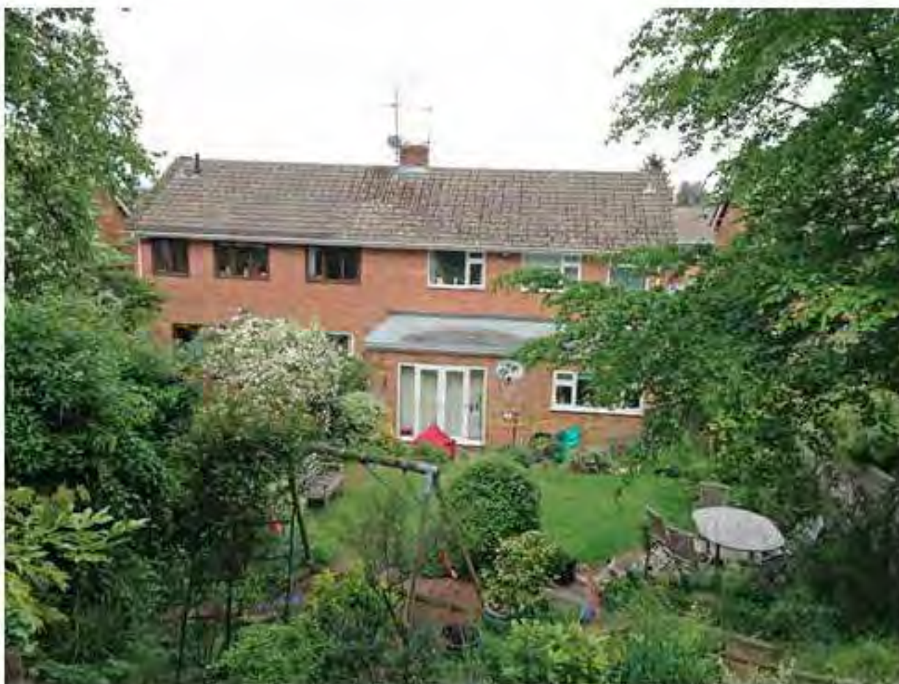
Eye level view from top of rear garden at 55 Collum End Rise
